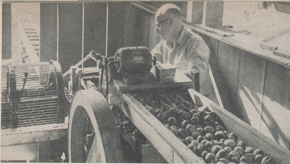
As the first step in processing the walnuts, Harry runs a crop through a hulling machine in his shed which uses a system of brushes and steel blades to scrape off the tough walnut hulls.
