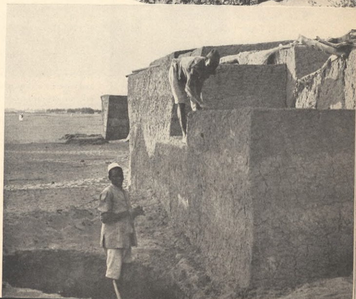
(Right) Mud and the sun form both walls and roof of houses built in the Egyptian desert
