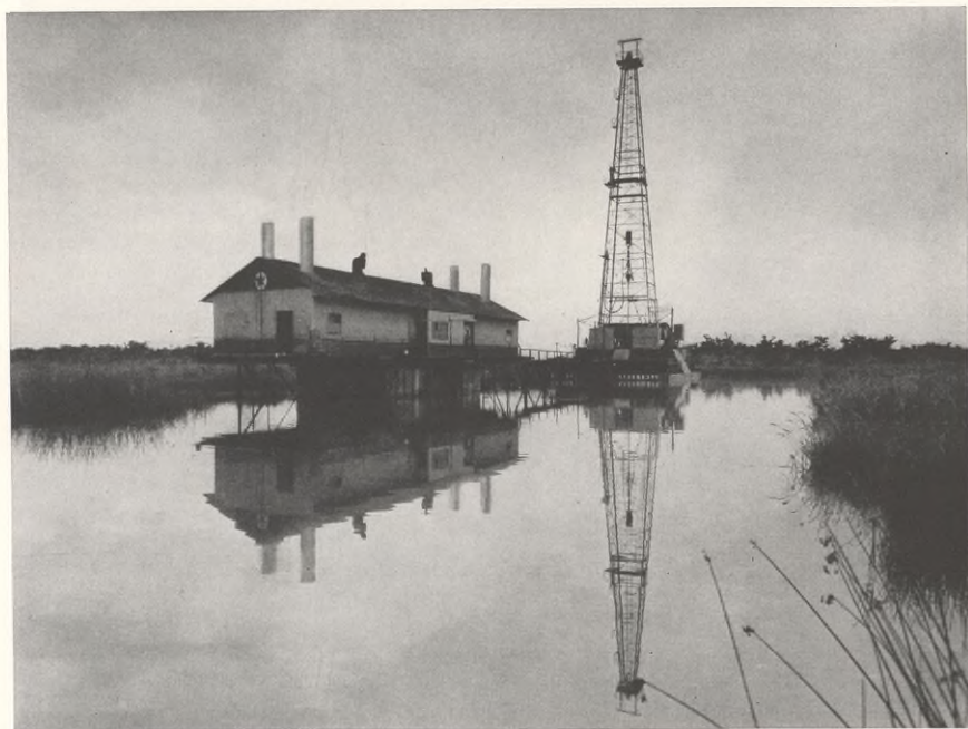
A Texaco-patented submersible drilling barge is towed to the site where a well is to be drilled, the lower compartment
