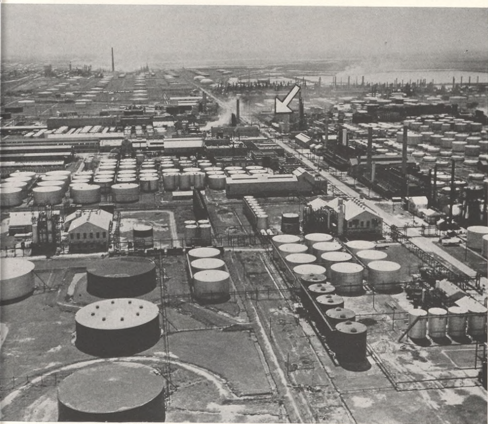
The arrow shows No. 1 Boiler House, almost lost in the midst of the tremendous plant which has been built up around it in four decades
