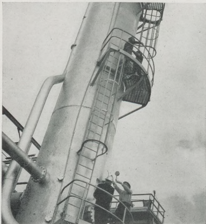
Revisions of equipment design, as in the fractionating tower at Houston (above), helped to raise Shell's daily average for refinery intakes by 5.4 per cent over that of the previous twelve months.
