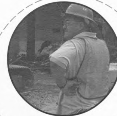
This construction foreman oversees the deconstruction of the library as his crew tears it down. Nathan Landsbaum
