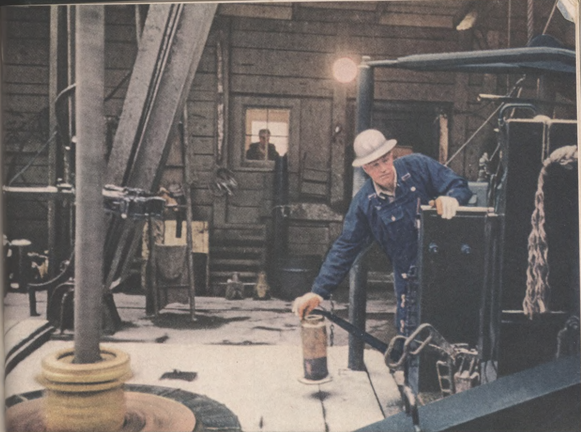
At Nig Creek, in northeastern British Columbia, the driller on a wildcat crew "runs the show." The brake lever is one of the numerous controls that demand his careful attention.
