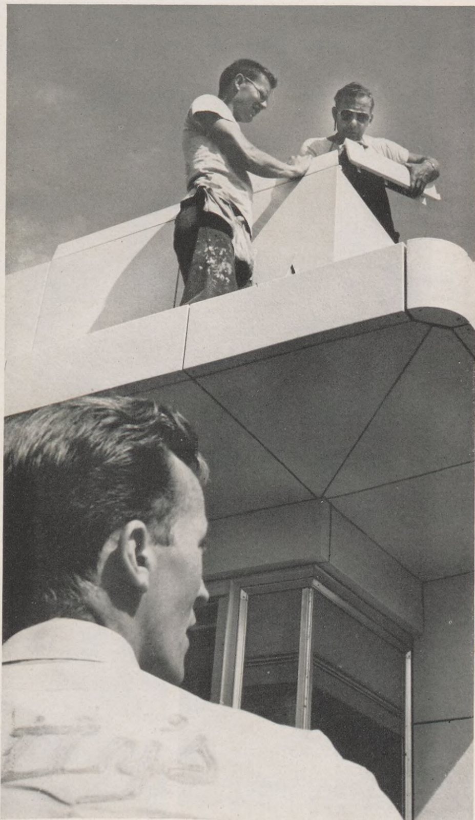
Scotty watches the porcelain trim being applied to the facade of his new station. These experienced workmen specialize in Shell's exclusive design and architecture. Throughout the construction period, Shell men were on hand to offer suggestions and advice.
