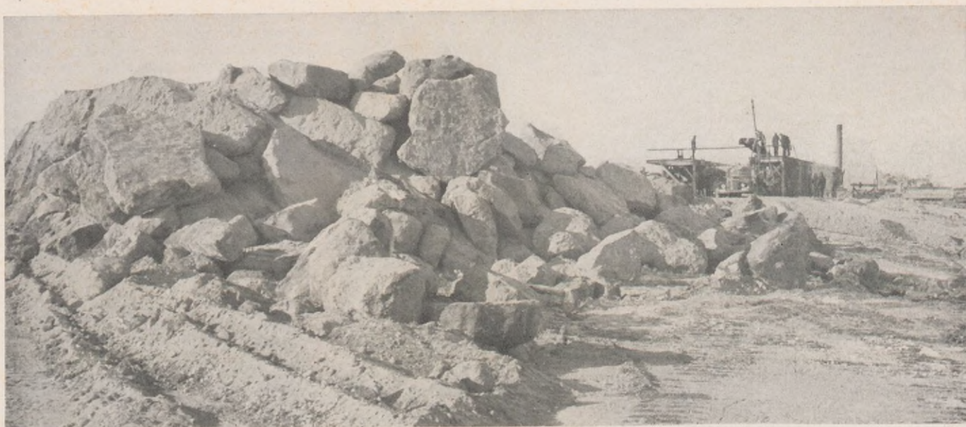
This is not a rock pile on the plains of northeastern Montana, but great chunks of frozen earth pushed up by bulldozers grading the location for a new Shell well in the Glendive Field not far from the North Dakota line. The blocks of rock-hard earth are from 36 to 48 inches thick.
