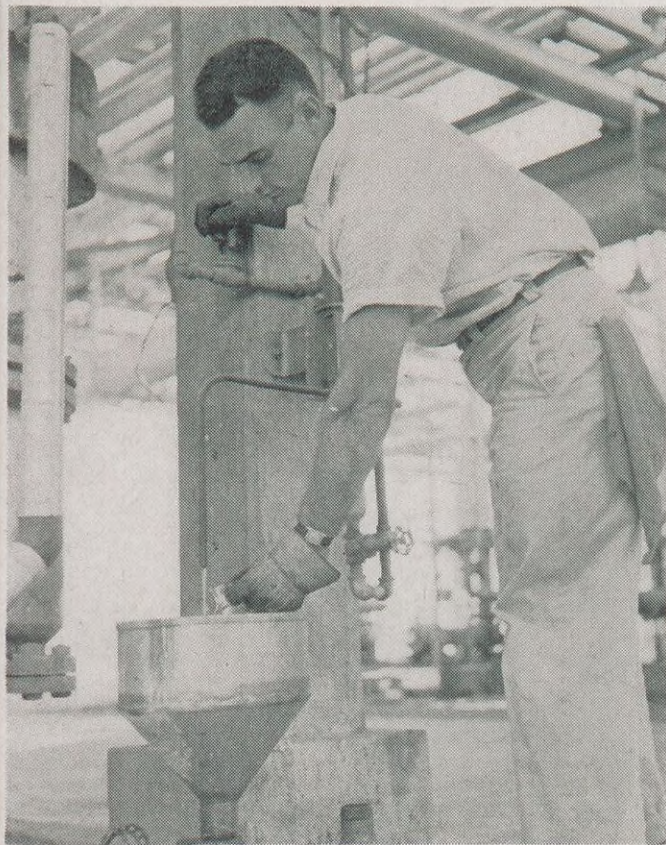
As the bringup proceeds, products are constantly checked and rechecked until they come up to specifications. Above, Operator L. E. Owens draws a sample of distillate for testing.
