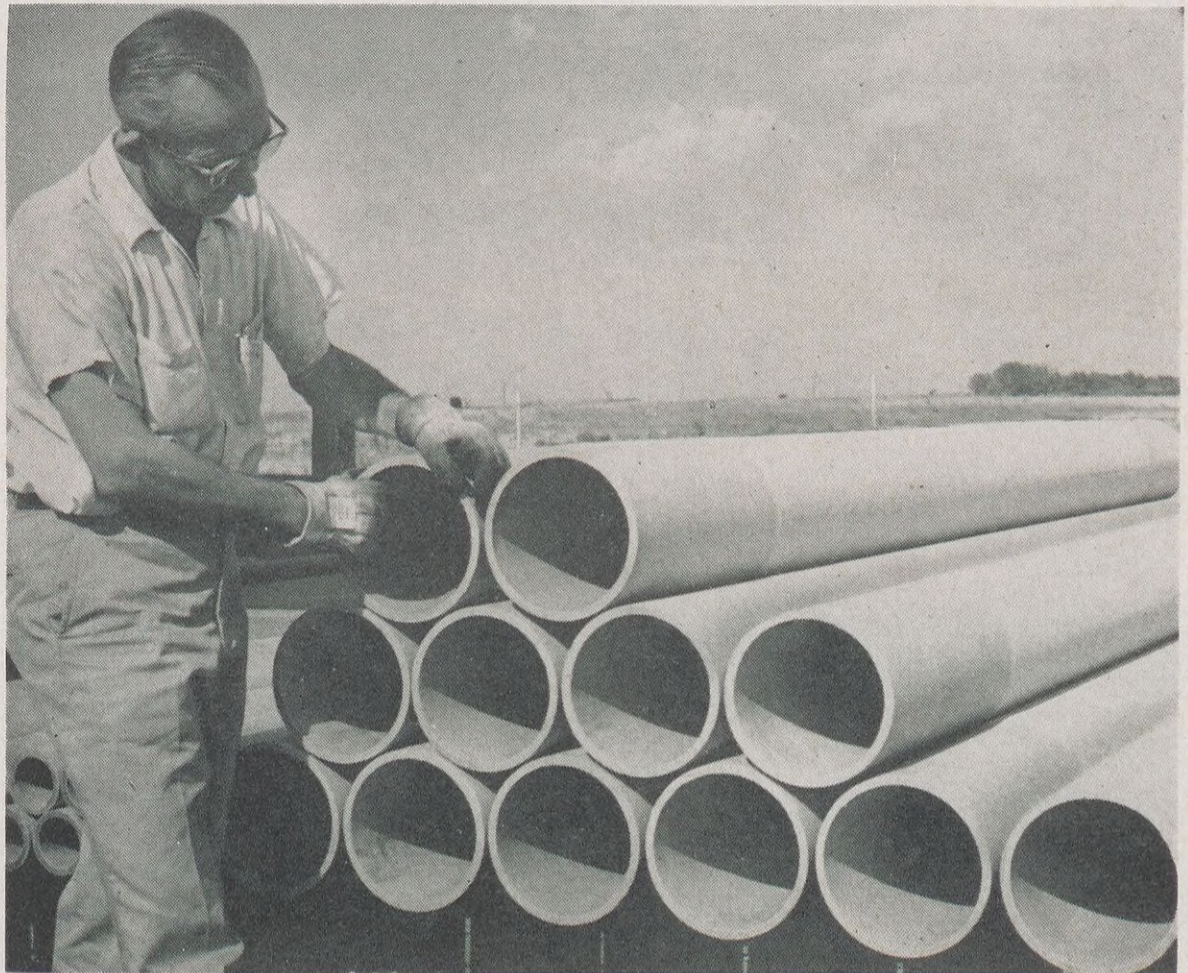
Salt water produced with Kansas crude necessitates non-corrosive piping. Above, Salt Water Disposal Operator W. A. Polley checks new pipe.
