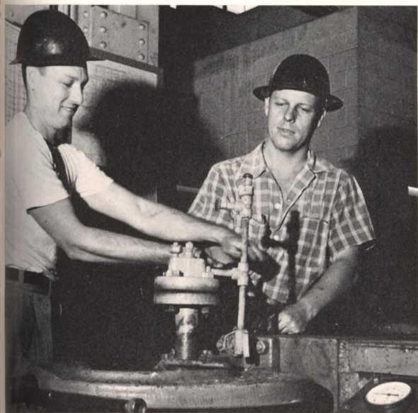
C. A. Janac, left, and W. A. Stabs repair a flow meter, one of Instrumentman's many duties.
