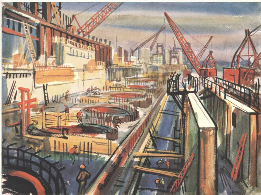
View from U. S. to Canadian side of St. Lawrence power dam. Shown under construction is line of 32 turbine-generators, 16 on each side of international border.
