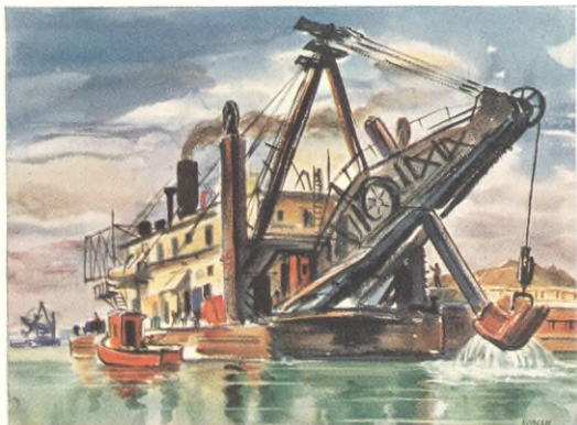
Bucket dredging at Lake St. Louis on the St. Lawrence is typical of great dredging operations needed to create 27-foot-deep channel.
