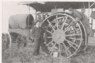
Engineer-Salesman H. D. Gohlman, Jr. demonstrating application of Crater Compound to tractors on the King Ranch near Kingsville, Texas
