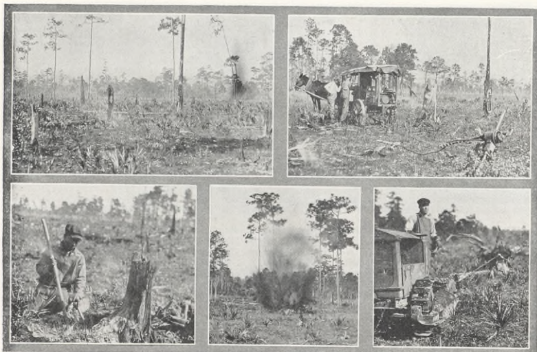
1. Land covered with stumps. 2. Mule wagon carrying a gasoline motor directly connected with an electric generator, which supplies the power for the motor in the drill shown in the foreground. 3. The man knows from experience how much Hercules powder to use, depending on the size of the stump. 4. The explosion loosens the stump from the lateral roots which spread in all directions. 5. After the shot it is generally necessary to pull the loosened stump from the ground by means of the tractor.
