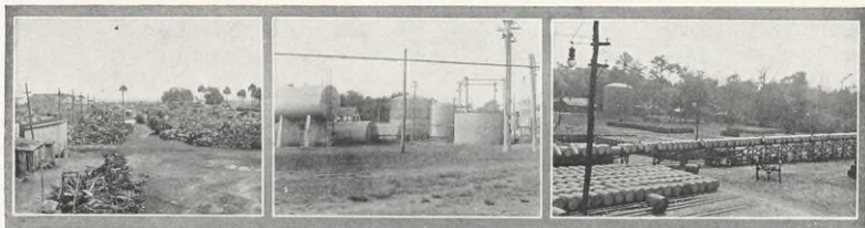
1. A supply of wood sufficient to run the plant for five weeks—about 15,000 tons—is kept in the wood yard at all times. 2. Part of yard tanks where liquid products are stored. Note the gasometer at the right. 3. Barrel runway from cooperage shop to rosin shed. In the background is seen one of the large storage tanks. In the left foreground is a shipment of rosin in barrels waiting to be weighed and loaded.
