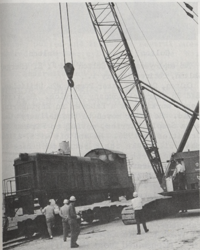
The 100-ton No. 1 Locomotive was lifted off the two wheel trucks so that traction motors could be inspected.
