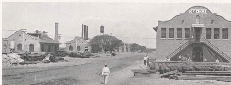
Tampico Works—looking west—Ice plant and electric power house in left foreground with boiler house and shops in the rear—End view of Office at right.
