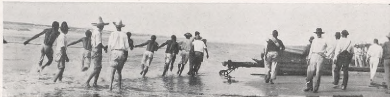
Attaching hawser for pulling Agua Dulce lines out to sea.
