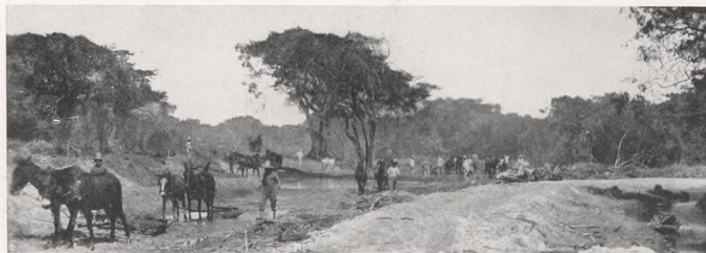
Clearing the property for Agua Dulce Works.
