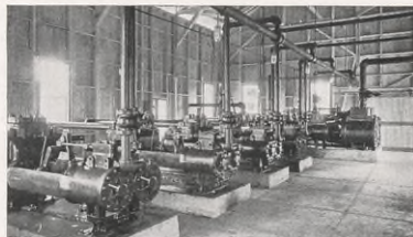
In the pump house at Tepetate Station.
