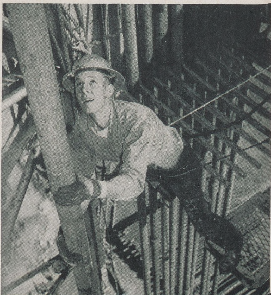
Joe steadies the long drilling string from above while other employees on the rig floor far below him handle the lower end. Additional sections of drilling string can be seen in the racks behind Joe. Each weighs about one ton.
