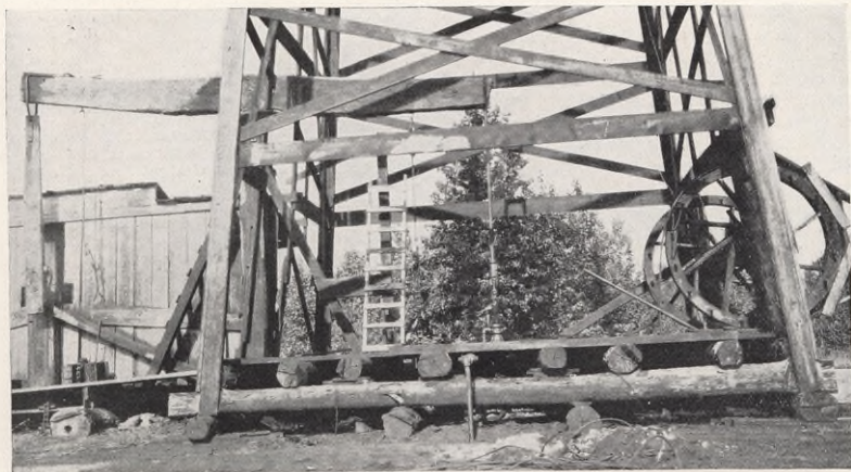
Well operated by engine whose walking beam operates two other wells
