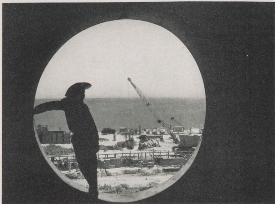
At the Cardon, Venezuela, refinery site (below), the combination of location and climate made the going rough for Shell construction employees.
