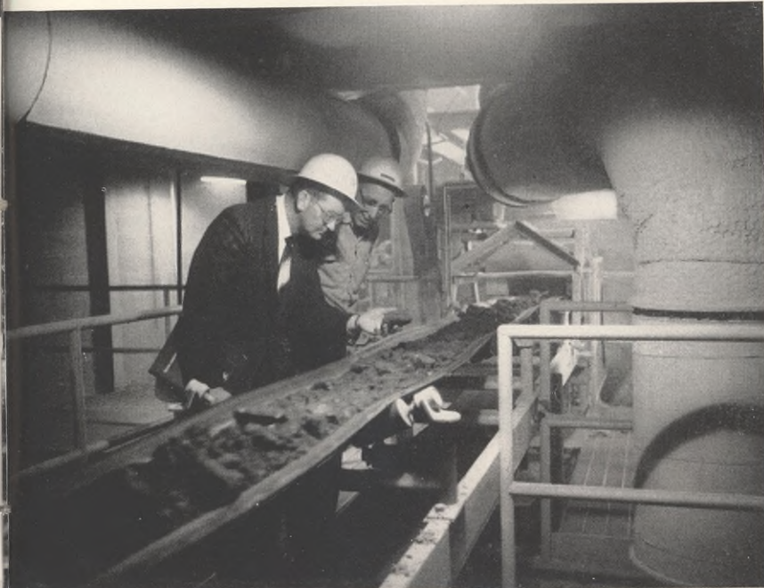
Conveyor belt, left, carries ore into the mill. After crushing, dye is assayed to determine uranium and vanadium content, which establishes market value.
