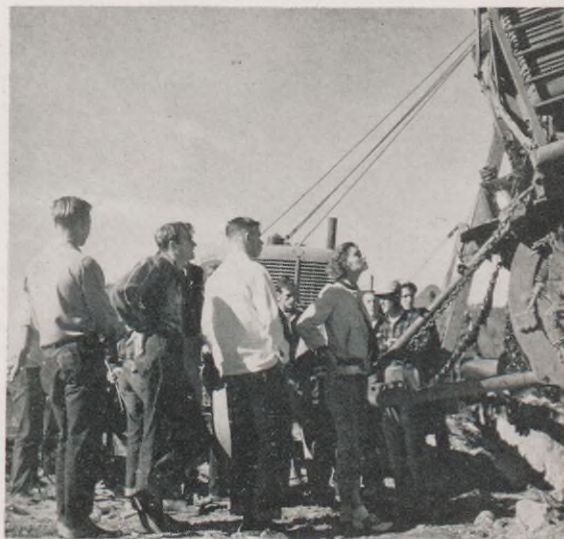
A Fredericksburg, Texas high school class visited the Rancho Pipe Line recently to get a first hand picture of pipe line construction.
