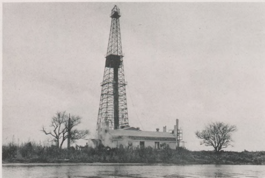
This rig drilled Shell's well at Weeks Island and recaptured the world's producing depth record.
