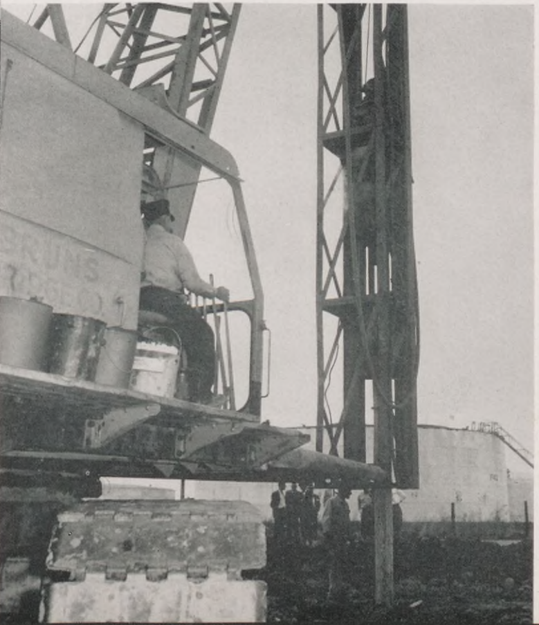
The first step involved in driving the trees into the ground at the Refinery is to fasten a steel plate on the butt end of each pile, left. This plate—later removed—keeps the pile from splintering under the pounding of the hammer. The pile driver, top, then lifts the pile into the hammer groove.
