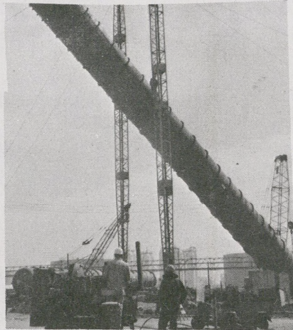
This column going up...the first of two 180 feet by 15 feet diameter columns was erected
