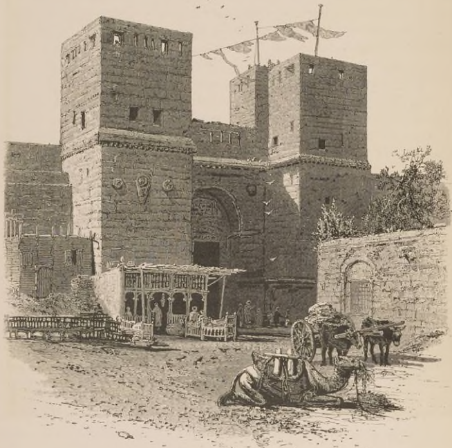
THE GATE OF VICTORY (BÂ'EN-NASR).
