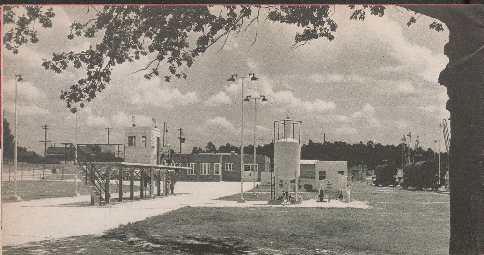
A Shell station on the Plantation Pipe Line near Doraville, Georgia. In the center is a calibrating machine and manifold, on the right, tank-cars ready to be loaded; on the left, a loading-rack for trucks; in the rear, the laboratory. Shell is one of the companies operating the line.
