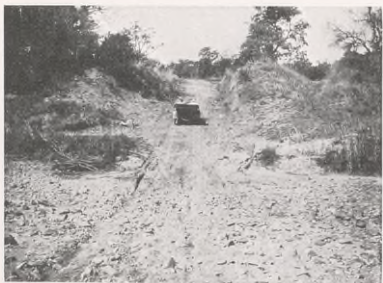
Sand and stones and steep gradient at the Que Que River drift
