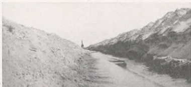
Canal constructed with this dredge—The canal is 10 feet deep and 45 feet wide at the top
