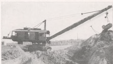
Dredge at work
