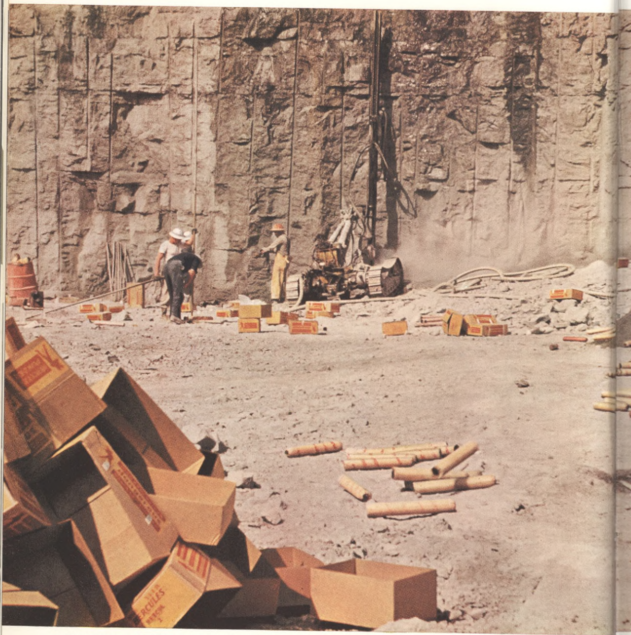
After tractor-mounted drilling rigs dig holes for dynamite charges to blast out beds for the giant conduits, crew inserts charges, tamps them down
