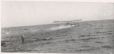
Hydroplane 183 leaving the water on its homeward flight. A speed of 42 miles an hour is necessary before it can leave the water
