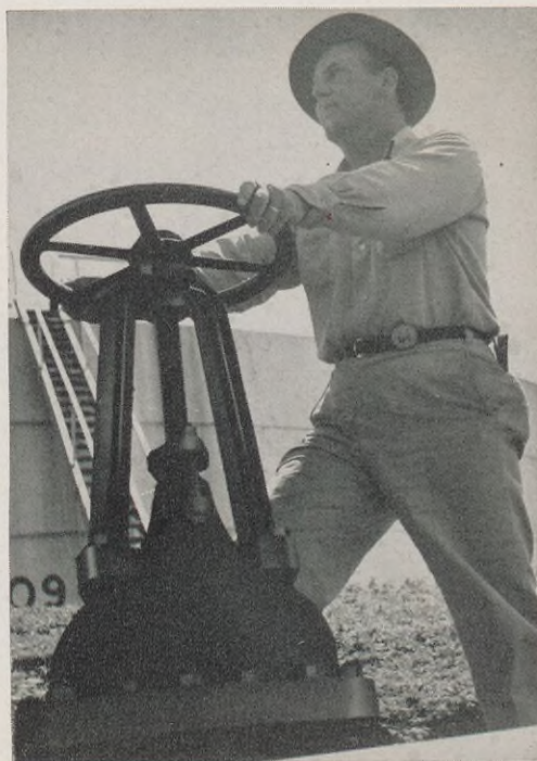
4. The Dispatching Department immediately readies a tank to receive the crude. Here Gauger A. F. Chaisson opens a valve connecting the tank with a pipe line from the unloading dock on the river.
