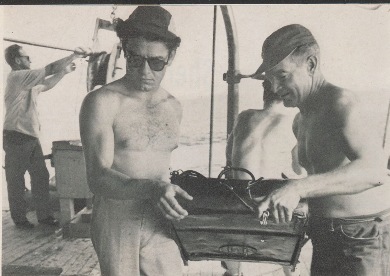
11. As each geophone returns to the instrument boat, above, the cable reel is stopped and the geophone is detached. The instrument is carried forward and lashed down for the night.
