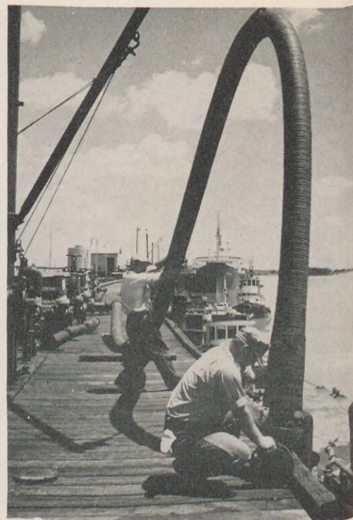
8. Guidry and Dock Helper H. J. Waguespack await a signal to lower an 8-inch hose to a barge outlet. A steam winch does the work.
