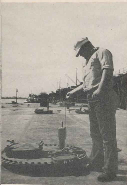
6. Each compartment of each barge is gauged by Guidry with a metal measuring tape and the figure is marked on the hatch with chalk.
