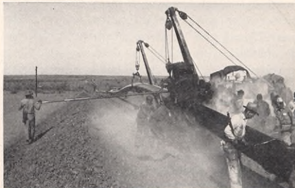
WRAPPING it up after cleaning and coating, pipeliners lower pipe into ditch, then backfill to cover the line
