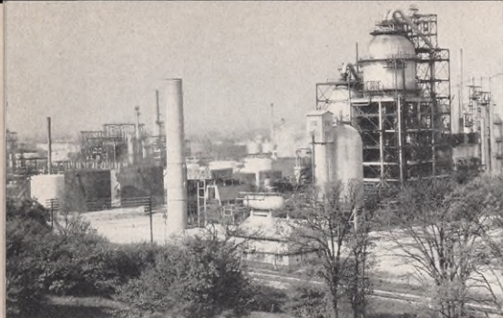
MAKING premium gasoline calls for refining facilities such as "cat" cracker (right) at Texaco's Lockport Works
