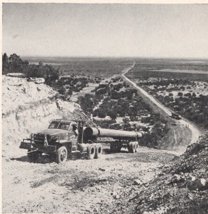
ROLLING their own, pipeliners truck pipe sections up a grade on the way from the railroad siding to location
