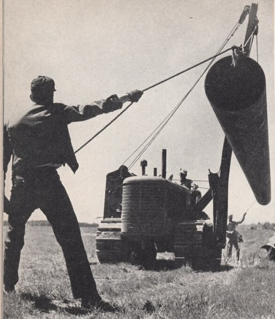
STRINGING them along surveyed route, "side boom cats" maneuver Basin-Ozark pipe sections into place
