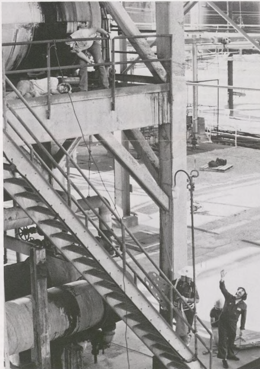
In a recent SMART drill, members simulated emergency medical and rescue procedures. Here J.D. Manning (top left) acts as the victim while Bubba Jackson (top right) prepares the stretcher hoist. Climbing the stairs with the stretcher is J.D. Young while Mike Rouse (standing) and Howard Lede prepare the equipment on the ground.
