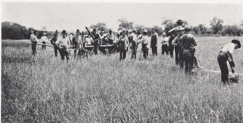
Laying 8-inch pipe near Dallas.
