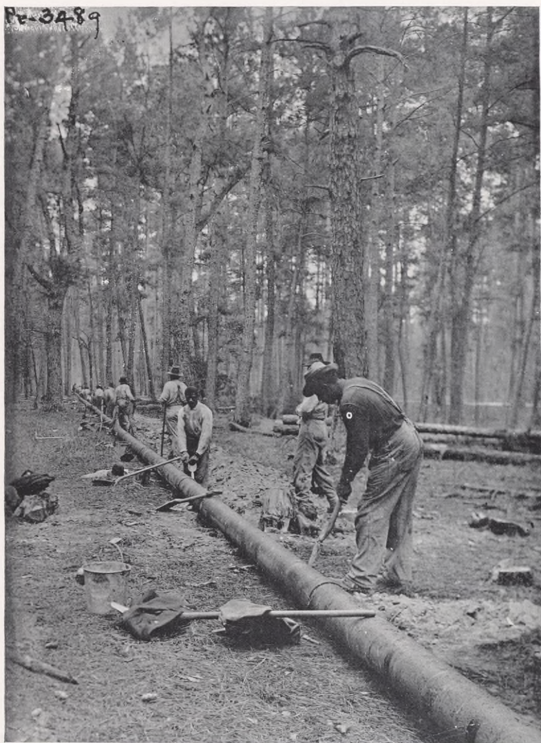
Ditching 8-inch pipe line in the piney woods of Texas.
