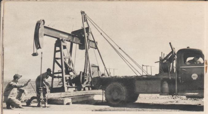
Setting a portable pumping unit at H. M. Sellens No. 1—typical of Shell's newer Western Kansas operations. These units serve three wells and are moved from location to location once each month. After the allowed production has been obtained from one well, the unit is disconnected, transferred to the next location in the manner shown, and reconnected. The entire operation requires approximately thirty minutes. From left: O. E. Houser, C. R. Warner, and H. J. Best.
