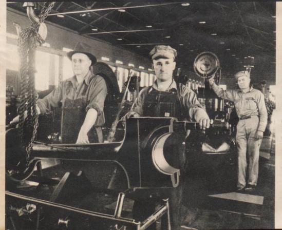
Shell Pipe Liners at work at Oetters Station. From left: H. R. Terrill, mechanical maintenance supervisor; E. A. Phenix, assistant mechanical supervisor, and J. W. Parks, mechanical maintenance supervisor in charge of automotive control equipment. **Terrill and Phenix** have just removed a piston from one of the engines, while Parks is examining an automatic regulator.
