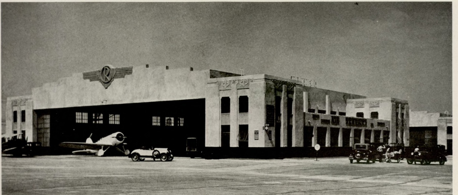
DETAIL OF HANGAR, ROOSEVELT FIELD, L. I.
