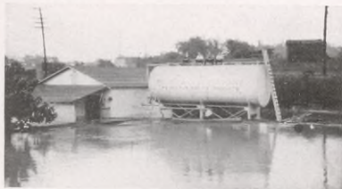
Rome, Ga. Station during the recent unprecedented flood
