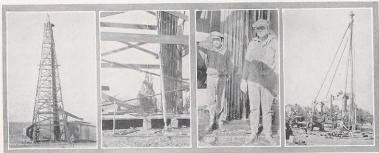
1. T. T. Co. J. F. Kenedy Well No. 4, Breckenridge Pool, flowing during clean-out operation, Nov. 18, 1924. 2. Same day: Well making a flow when tools were being removed from hole. 3. T. T. Co. J. W. Parks Well A 31, Breckenridge Pool—a clean-out crew, Nov. 18, 1924. 4. Drilling equipment for shallow wells in Moran Pool—good for about 800 feet.
