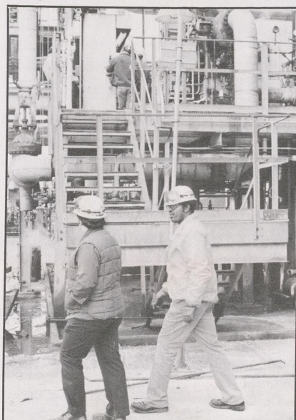
Operations foreman Danny Mills (l) and Paris Reescano helped coordinate construction and operations related to new Selective Hydrocracker.
