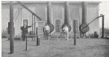
North Side of Berwick Fuel Oil Station
