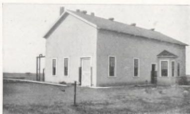
Fuel Oil Terminal Station, Berwick, La.
