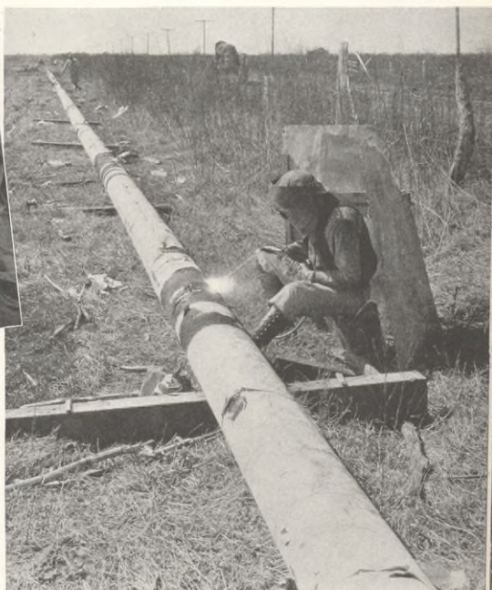
(Right) On some lines the ends of pipe are joined by welding. When this welder finishes his work, the pipe line will be lowered into the ditch which has been dug for it
