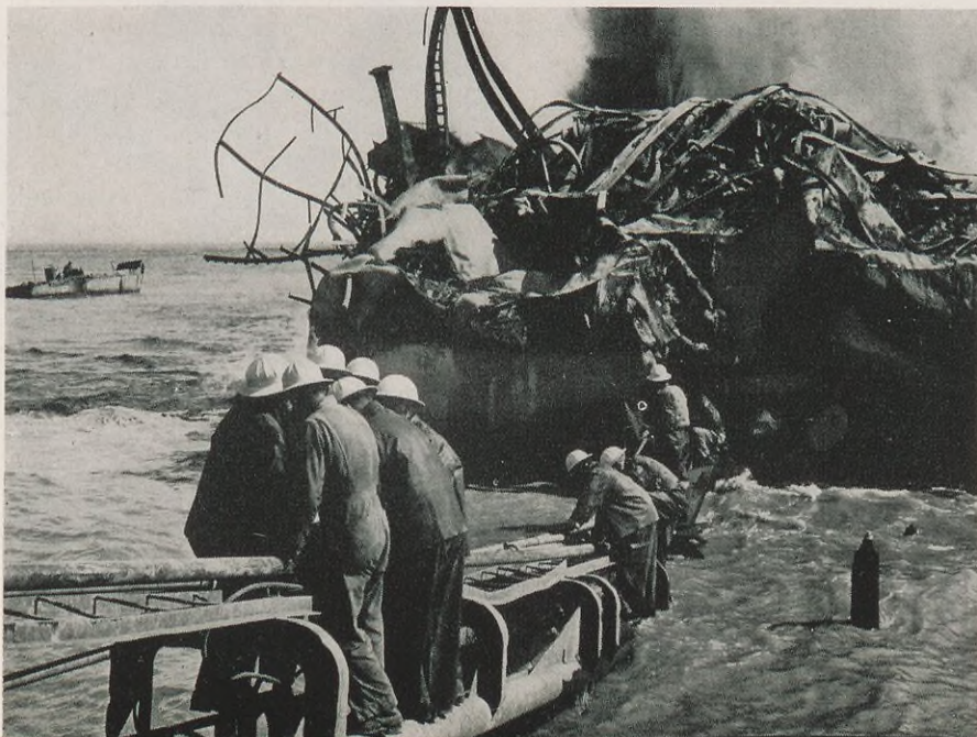
The melted derrick crashed across a tank battery, above, adding more fuel to the fire, which raged 22 days. At left a crew runs lines to seal Well No. 1 with cement. The drilling barge and two LSM's disappeared in the crater the fire caused.
