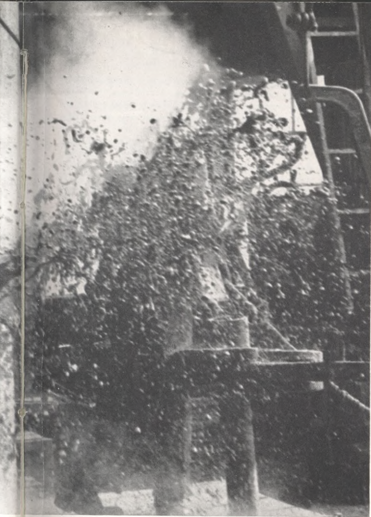
Breaking "stem," or drill pipe, aboard the barge Gibbens, left, roughnecks wait for excess water and mud to run off — a standard procedure in the early stages of tidelands drilling. The intent driller, above, is responsible for all activity on derrick floor.
