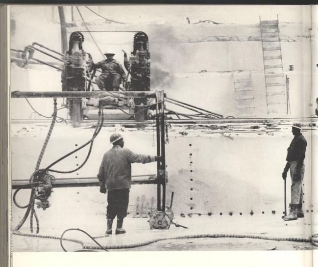
Channeling machines, above, cut 30-ton blocks of marble from the sides of a North Georgia quarry. Below, a Texaco lubrication engineer makes a service call at quarry bottom 100 feet down.
