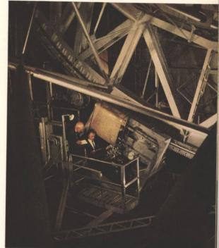
In the tracking mechanism, a Texaco lubrication engineer and a Telstar project technician review lubrication procedures for the pumping units on the antenna's hydraulic power systems.
