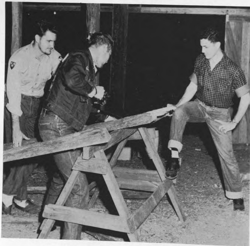
Don Leissner cuts slabbing for the Bella Union balcony . . .
