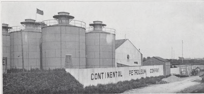
Antwerp, Belgium: Continental Petroleum Company's gasoline storage tanks.
