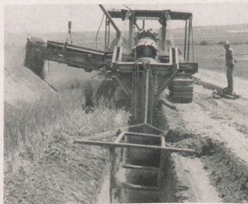
2. DITCHING: A ditch digging machine, below, cuts a five-foot deep trench across a prairie and not far behind a "stringing" crew, below left, drops lengths of pipe into place beside the ditch.
