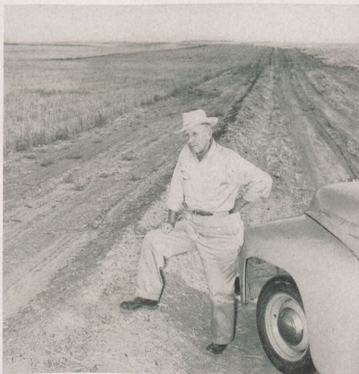
7. THIS IS A PIPE LINE: Only a long narrow mound of earth, above, indicates where ditchers, stringers, welders, wrappers and backfillers have passed. Beneath the mound, crude oil flows from oil fields to refineries. D. E. Rubottom, a clean-up inspector for Shell Pipe Line, looks over a completed section of line.
