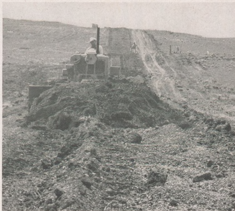
6. BACKFILLING: As the doping and wrapping machine moves along the pipe, the coating is inspected and the pipe is then lowered into the ditch, left. Bulldozers complete the construction cycle, left and above, pushing earth back into the ditch and smoothing the right-of-way. Foot-by-foot, mile-by-mile a new pipe line snakes its way beneath the soil of the states of Montana and Wyoming.
