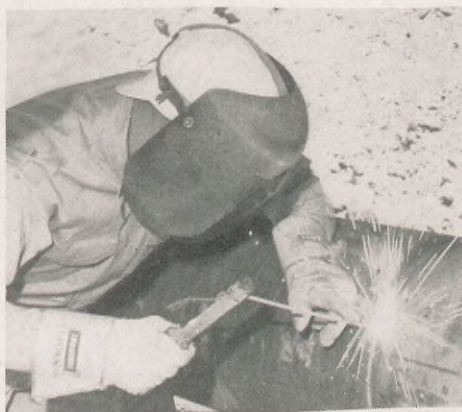
3. JOINING: Welding teams, above and right, follow the stringing crew, making one continuous line of the many shorter lengths.
