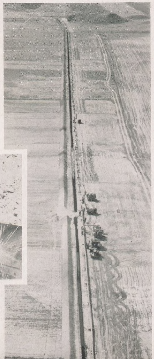
2. DITCHING: A ditch digging machine, below, cuts a five-foot deep trench across a prairie and not far behind a "stringing" crew, below left, drops lengths of pipe into place beside the ditch.
