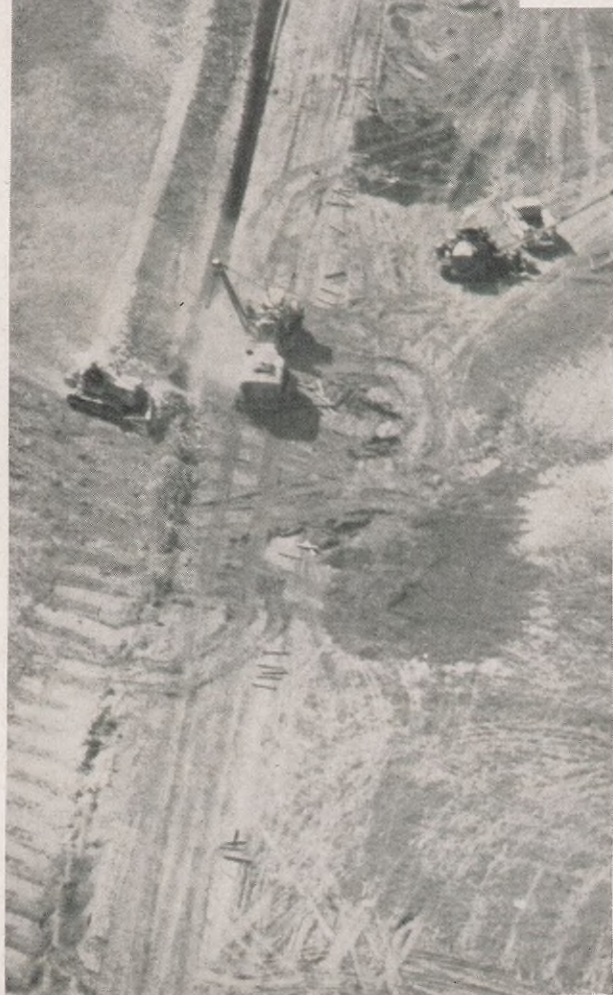
7. THIS IS A PIPE LINE: Only a long narrow mound of earth, above, indicates where ditchers, stringers, welders, wrappers and backfillers have passed. Beneath the mound, crude oil flows from oil fields to refineries. D. E. Rubottom, a clean-up inspector for Shell Pipe Line, looks over a completed section of line.
