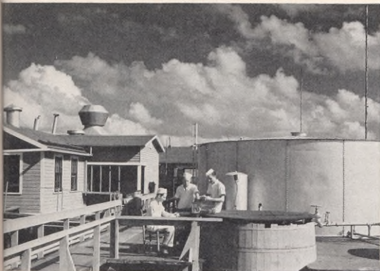
CAILLOU ISLAND —Peeling potatoes for supper at Caillou Island field camp are (l. to r.) H. M. Breaux, A. P. Naquin, and E. J. Breaux. Camp is built on piling
