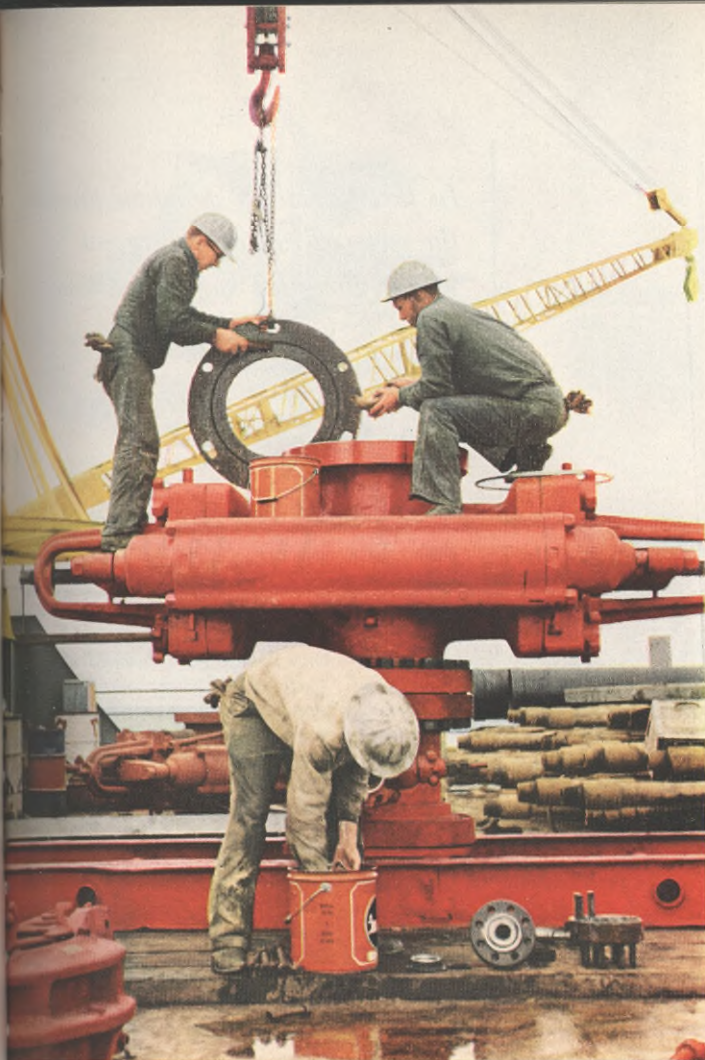
The elaborate mechanism for preventing a blowout of the well is readied for installation.
