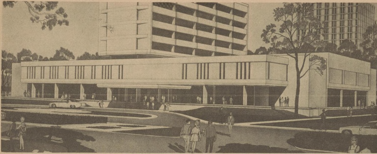
Center for continuing education and hotel and restaurant school
