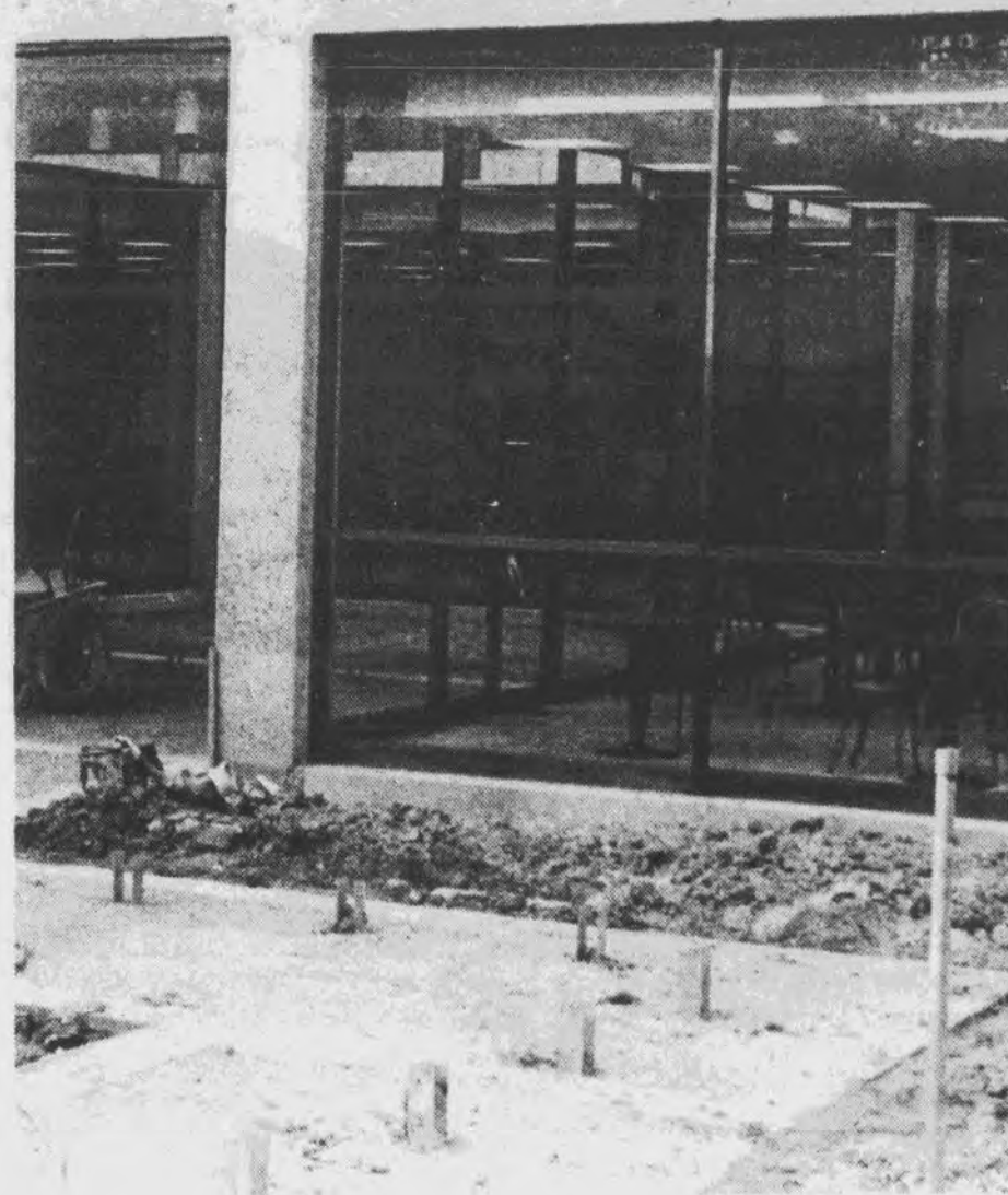
UC SATELLITE, sandwiched between the Science and Research Building and parking lot Number 5, opens Monday. One of the hidden aspects of the building is the fact that the building is somewhat hidden under the sidewalk.
