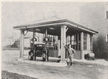
McAdoo Filling Station, Jersey City, N. J.
