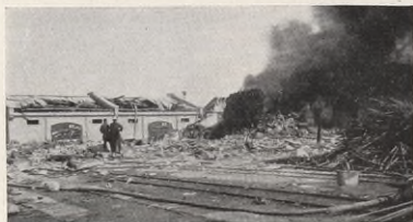
All that was left of our warehouse at Shantung, China
