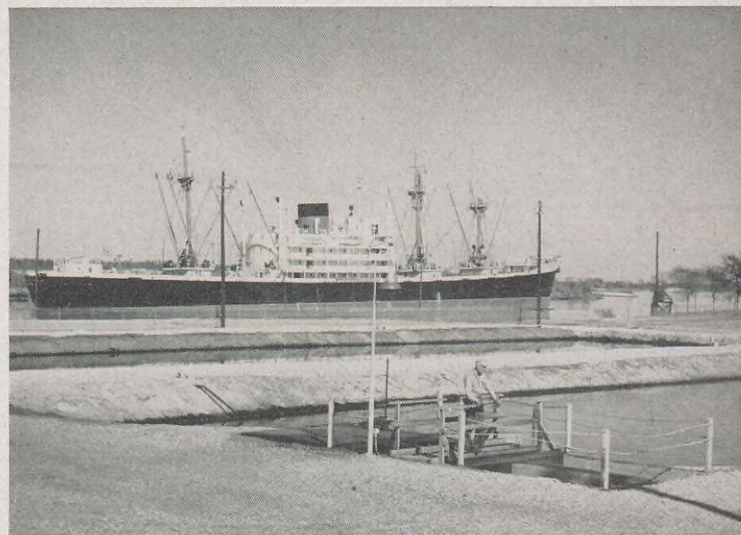
Above, A. P. Jackson, Pumper in the Refinery Effluent Control Department, operates equipment at an oil and water separating pond as a ship passes nearby on the Houston Ship Channel. Tiny bacteria in the pond consume particles of oil in the water.
