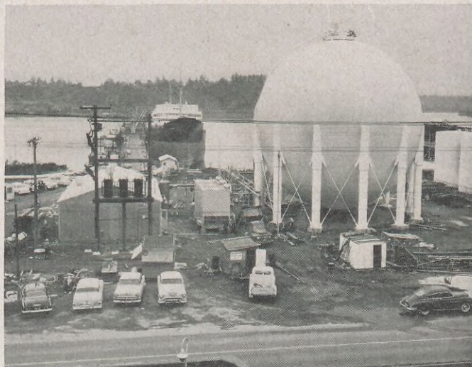
Here, the sphere has been covered with a sealing compound and painted white. Both the sphere and its compressor building, to the left of it, are completed. Shell's dock and a tanker are visible in the background.
