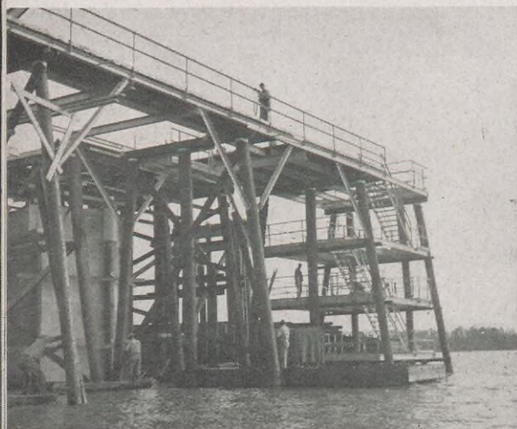
The 492-foot wharf, above, where barges and ships will be loaded and unloaded, provides four levels to allow for rise and fall of the Mississippi River. Pumps to provide water for the plant are housed near the end of the wharf.
