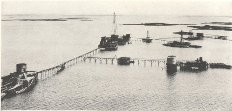
General View of Operations on a Water Location: Lake Barre Dome, Louisiana
