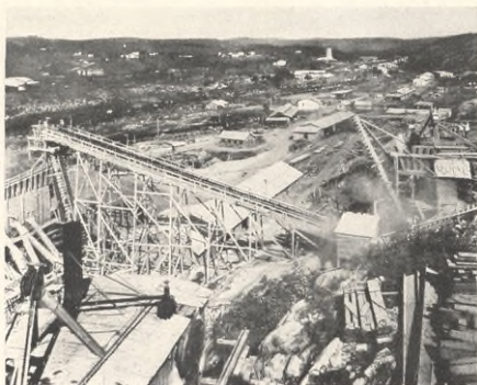
City of Bananeiras During Construction Work
