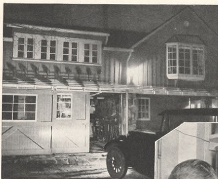
The Garage Doors Respond to the Flash of the Headlights
