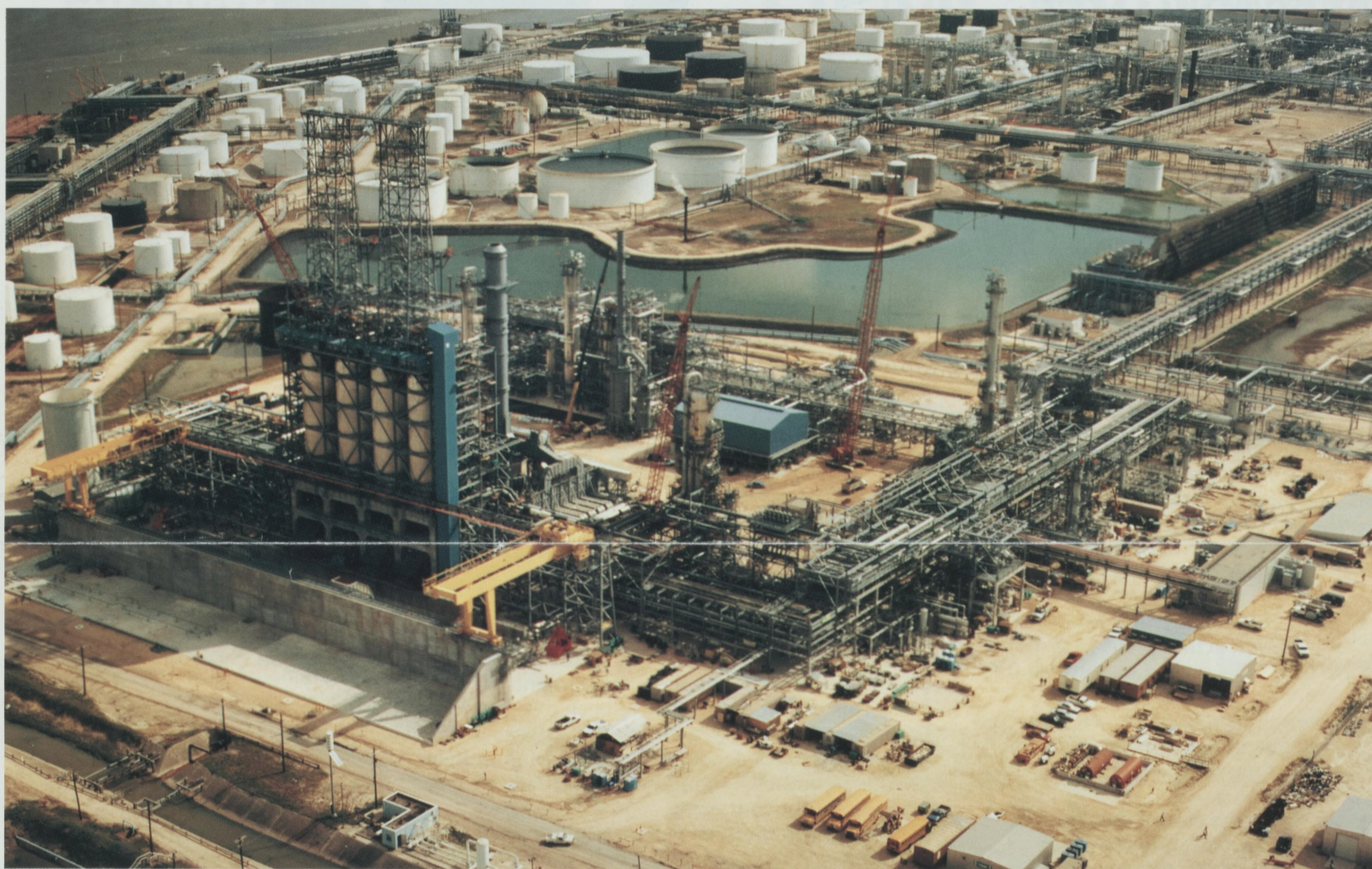
Aerial view of the delayed Coker Unit taken shortly before startup.
